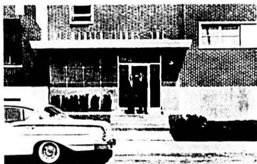
Delmonico Foods of Louisville has just completed a new addition of some 50,000 square feet. Pictured are President Peter J. Viviano and his son Joseph in front of the new office entrance on South Floyd Street.
