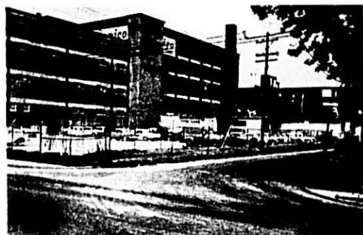
The four-story addition permits straight-line production with gravity feed from production departments to packaging and warehousing. The new section is to the left with the original structure on the right.
